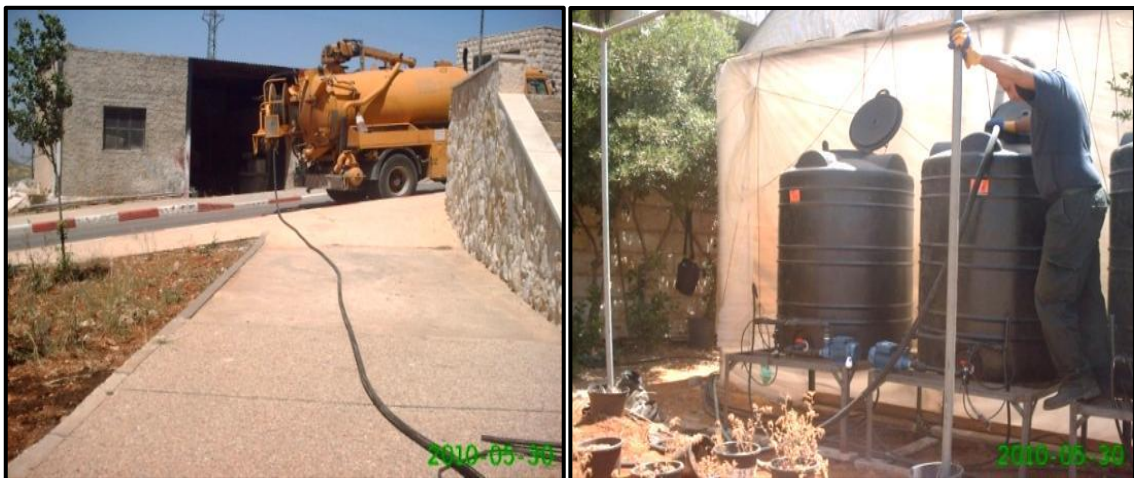
Figure (3.6) Transportation and Filling of TWW
